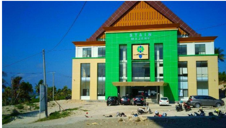
Gambar 4.1 Gedung STAIN Majene
