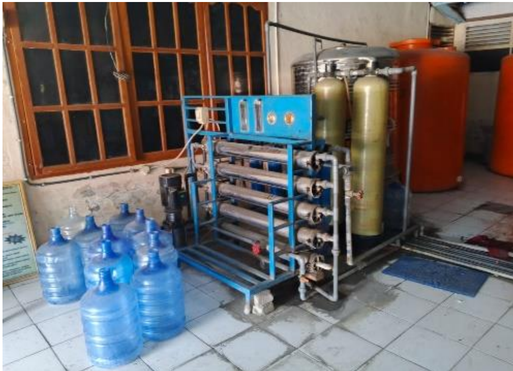
Gambar 4.1 Keadaan Filtrasi depot HL
